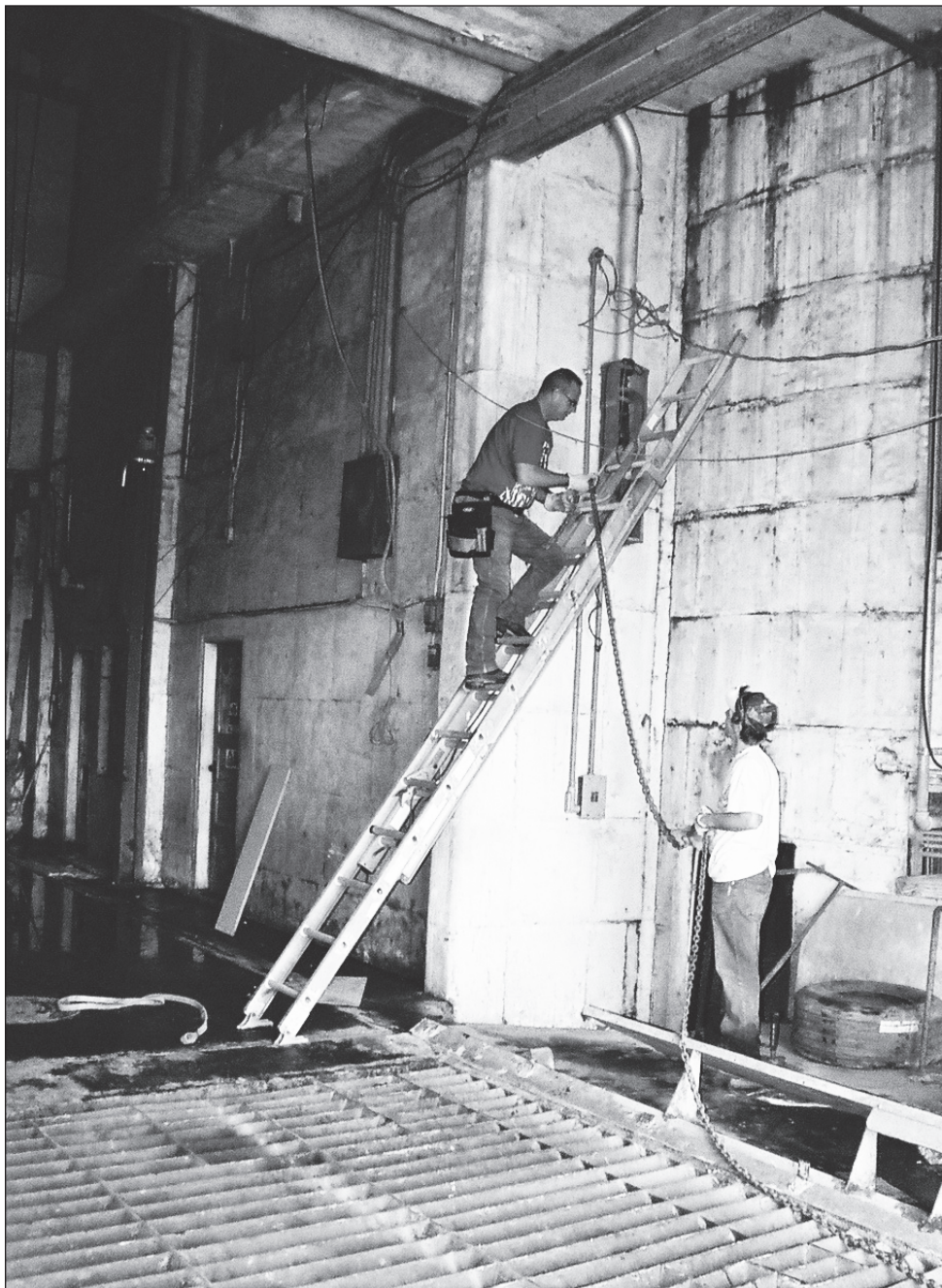
Crew members are removing recycleable wire and metal from the rice dryer. The grating is the dumping station where rice was dumped onto a conveyor to be carried to the actual dryer. This once state-of-the-art dryer only had the one dumping station which meant that many longtime Dayton residents have memories of rice trucks lined down the road at harvest time, waiting to dump their load. After the rice was dumped through this grating, it was then moved by conveyors to the necessary bin or dryer.
